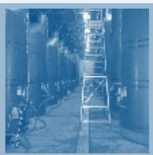
Boundary Bend processing plant
