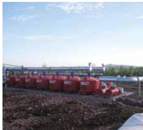
Sandalwood – pumping station.
